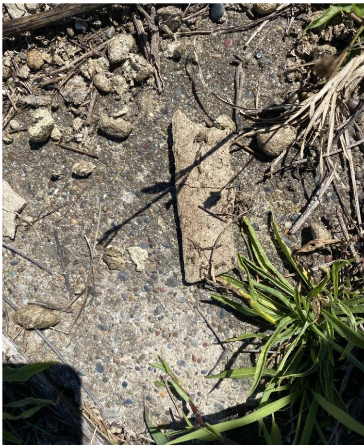
Photograph 12 - Loose ACM piece on old concrete slab.
